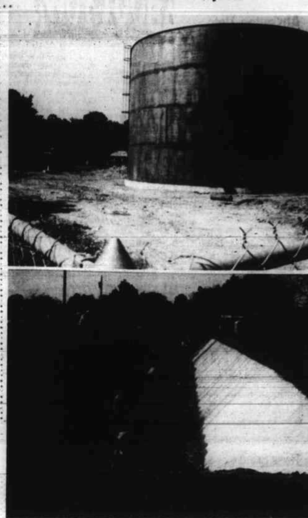
City's new 500,000 gallon water tank is being constructed at the new water plant site on Davitt Street (top photo); and the first concrete walls for the flood drainage ditch from the intersection of East Main along 4th Street south to the Eagle Lake Primary School, have been poured as seen in the lower photo.
